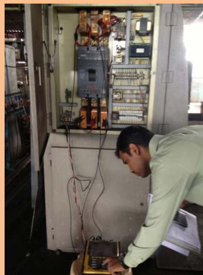
Field measurement during energy audit
