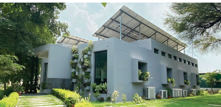
The Mahindra-TERI Centre of Excellence for Sustainable Habitats at Gurugram
