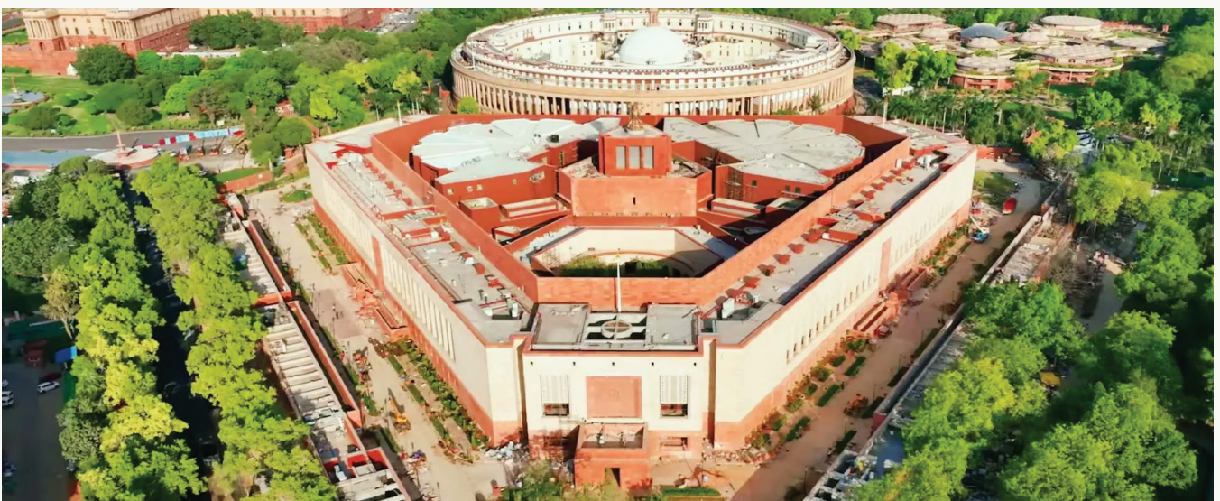
► The new Parliament building, under India's Central Vista Redevelopment Project, is registered with GRIHA and aspires to achieve a 5-star GRIHA rating
