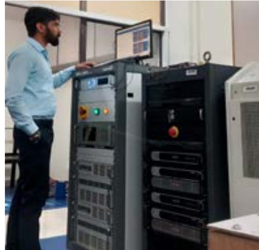
BESS pilot site visit by DST, IUSSTF, PMC team
