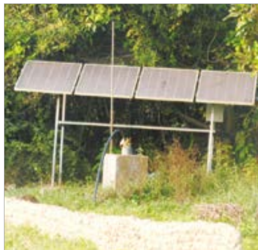
Solar-powered RBF well at Navelim, Goa
