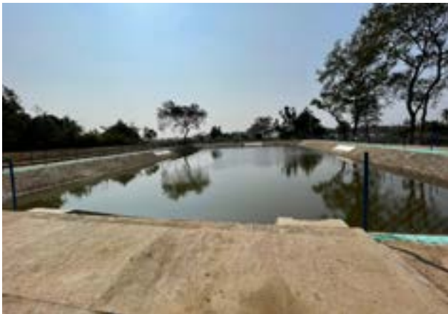
Water conservation through pond rejuvenation
