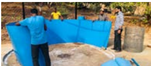
Installation of Biofloc unit at Mokhada, Palghar
