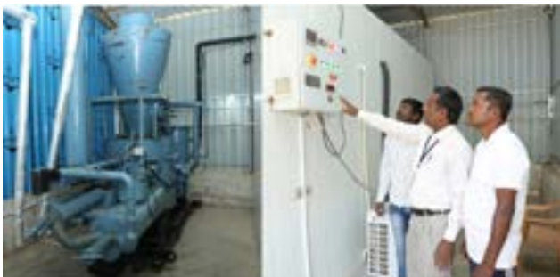
Vapour absorption-based cold storage operated with biomass gasifier
