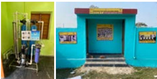
Drinking water and sanitation facility developed in schools
