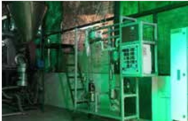
► Bio oil catalytic upgradation unit
