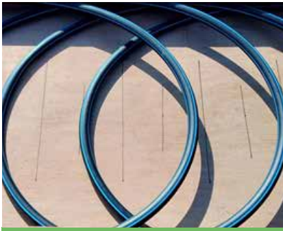
» Installation of geo-exchange loops
