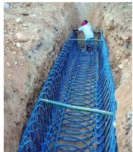
» Onsite fabrication of geothermal slinky
