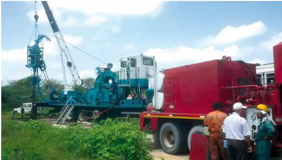
Field-scale implementation of PDB technology for enhanced oil recovery from oil reserves
