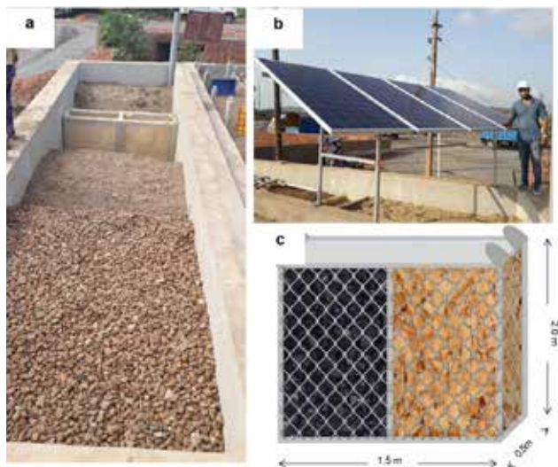
(a) The triangular horizontal river bed filtration tank with different filter materials and the anti-microbial cage; (b) Solar panels (used for powering the pump) mounted on the BF tank; (c) Design of the cage with antimicrobial material (silver impregnated activated charcoal (left) and wood shavings with TPA (right))
