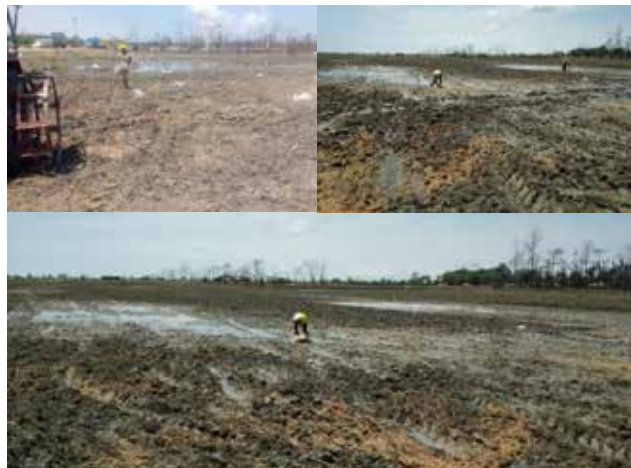
Application of microbes and tilling at the oil-contaminated site
