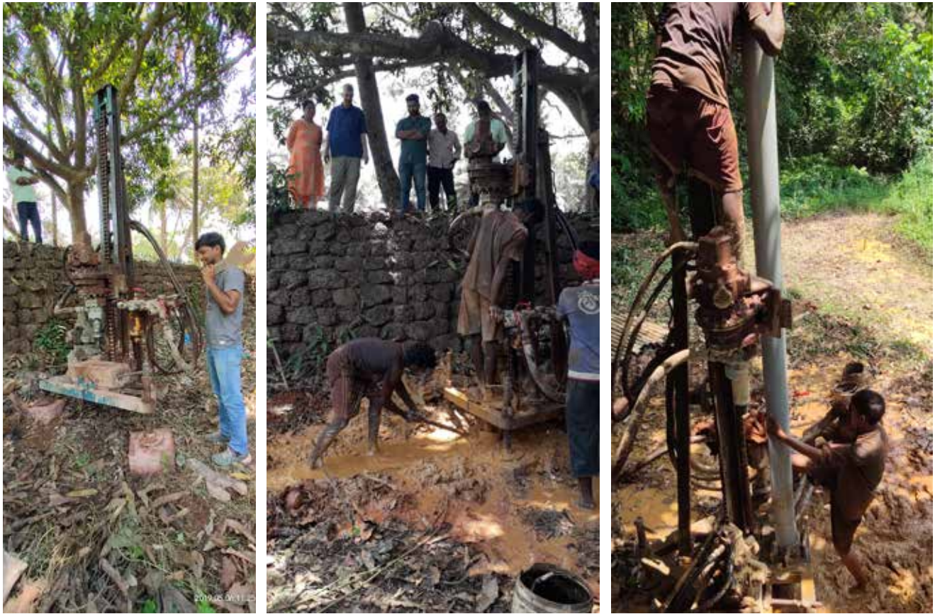
Drilling and installation of RBF wells at Cortalim
