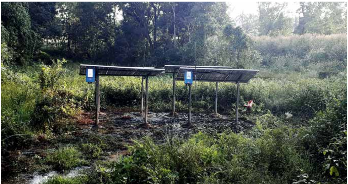
RBF solar panels installed for sustainable power supply for the functioning of the borewell pumps at Cortalim site
