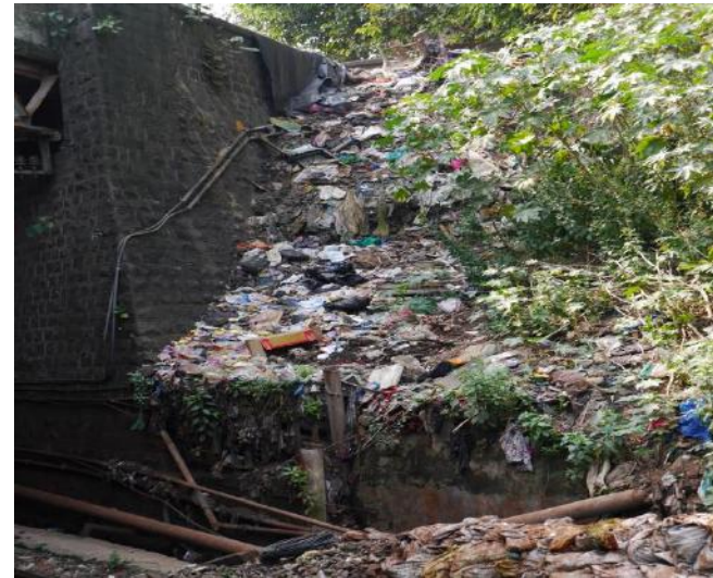
Along railway tracks and other leakage points
