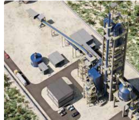
FLD Smith's Clay Calciner System
