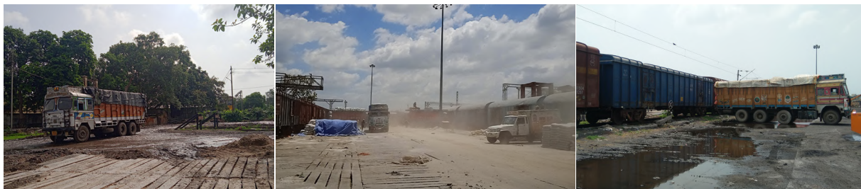
Figure 51: Poor wharf and circulation area
