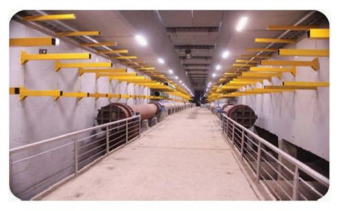
FIGURE 22 Utility tunnel, showing support brackets
