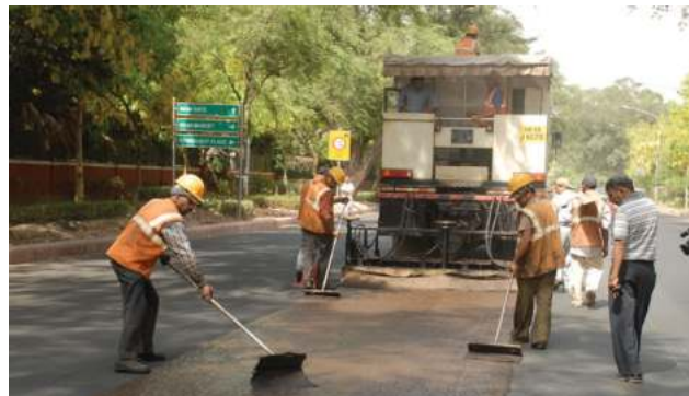
iv. NDMC roads are maintained for crack sealing and maintenance
