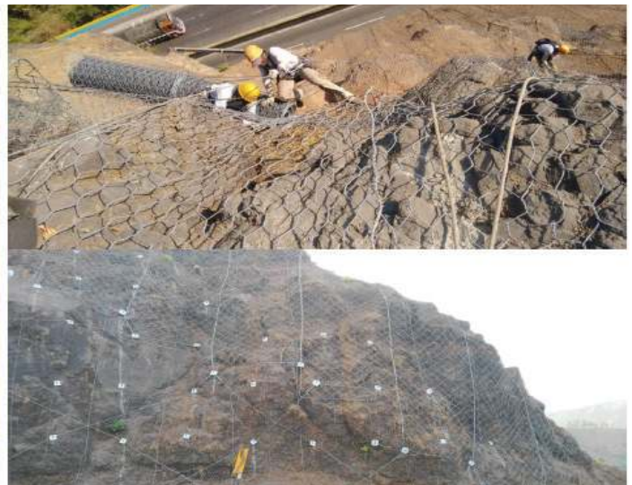
viii. Usage of mono oriented reinforced steel wire mesh, rhomboidal cable wire rope panels, dynamic rock fall barriers, anchors, Mumbai –Pune Expressway
