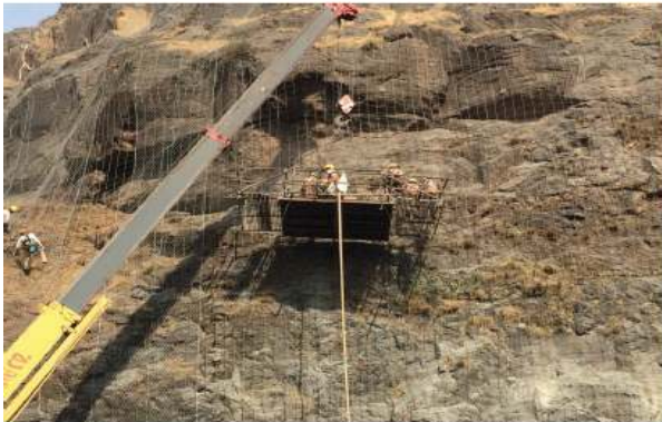
viii. Usage of mono oriented reinforced steel wire mesh, rhomboidal cable wire rope panels, dynamic rock fall barriers, anchors, Mumbai –Pune Expressway
