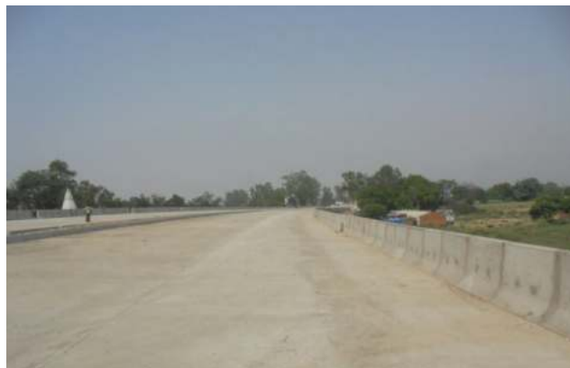
Photo 6: Pavement quality concrete work under the Etawah–Chakeri project (Source: NHAI)
