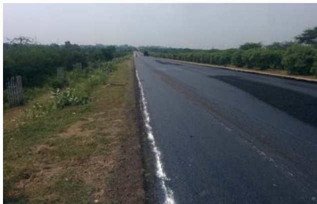
Photo 5: Overlying work on the Orai–Barah section of NH-25
