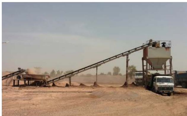
Photo 1: Crusher unit for the upgradation of the Jodhpur–Pokhran NH-114
