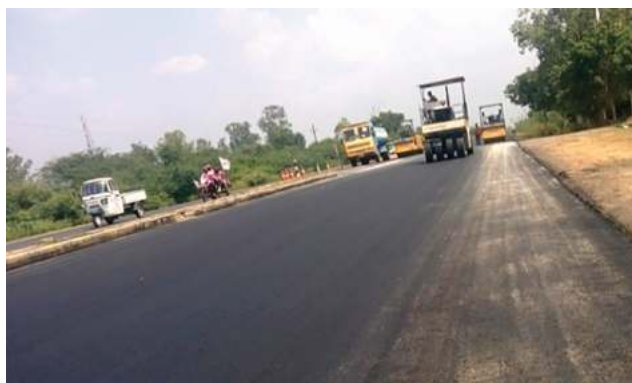
Figure 24: A photograph from the maintenance site
