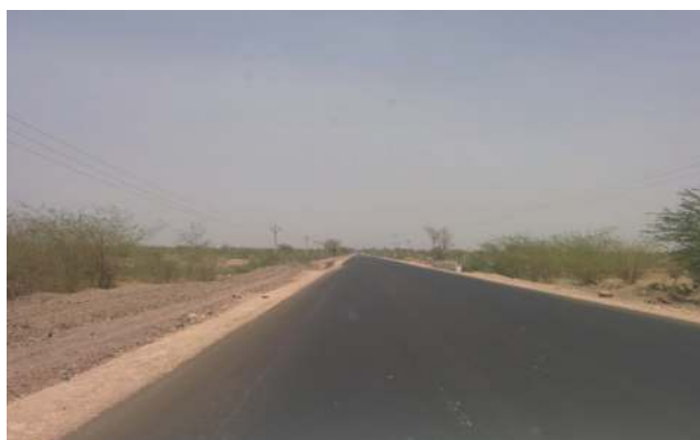
Photo 3: Expansion work under the Jodhpur–Pokhran section of NH-114
