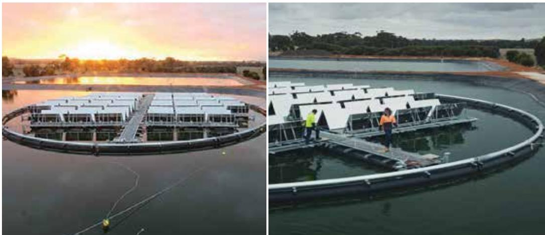
**Figure 12:** Phase I of 4MWp floating solar PV plant at wastewater treatment facility, Jamestown Australia
