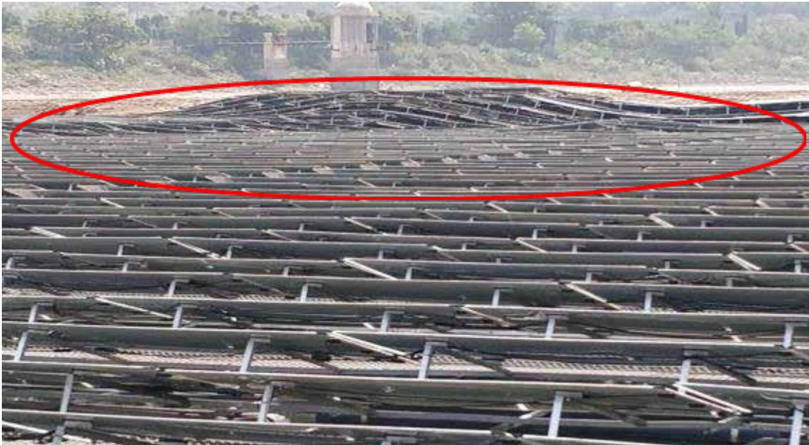
**Figure 21:** Impact of improper bathymetry and/or hydrography surveys
