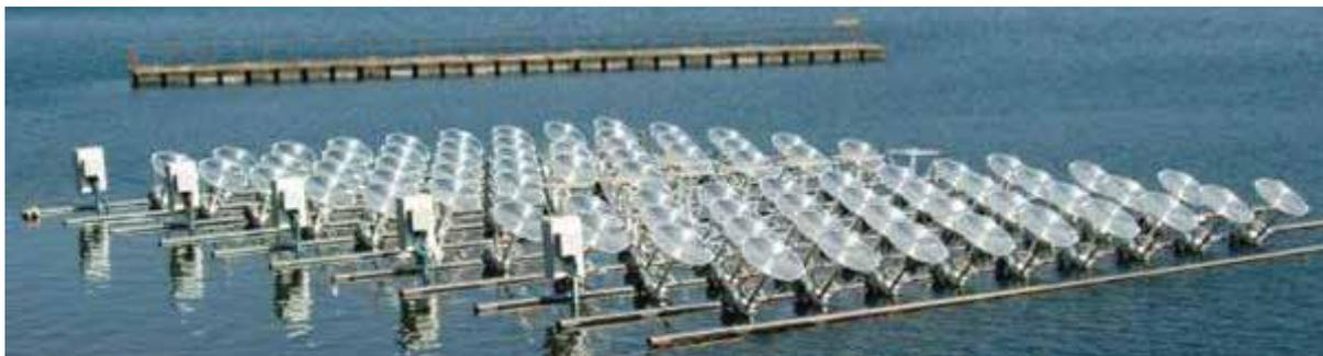
**Figure 14:** A pilot installation based on liquid solar array technology by Sunengy in hydro dam in India
