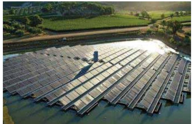
**Figure 10:** A-200 kWp grid-connected single axis based floating solar PV plant in Suvereto, Italy
