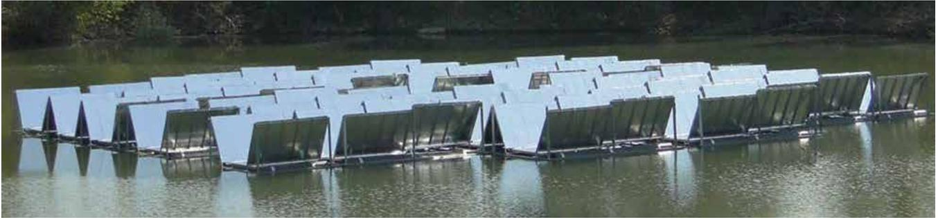
**Figure 13:** A pilot installation in Colignola (Pisa) on an artificial basin by Koine Multimedia
