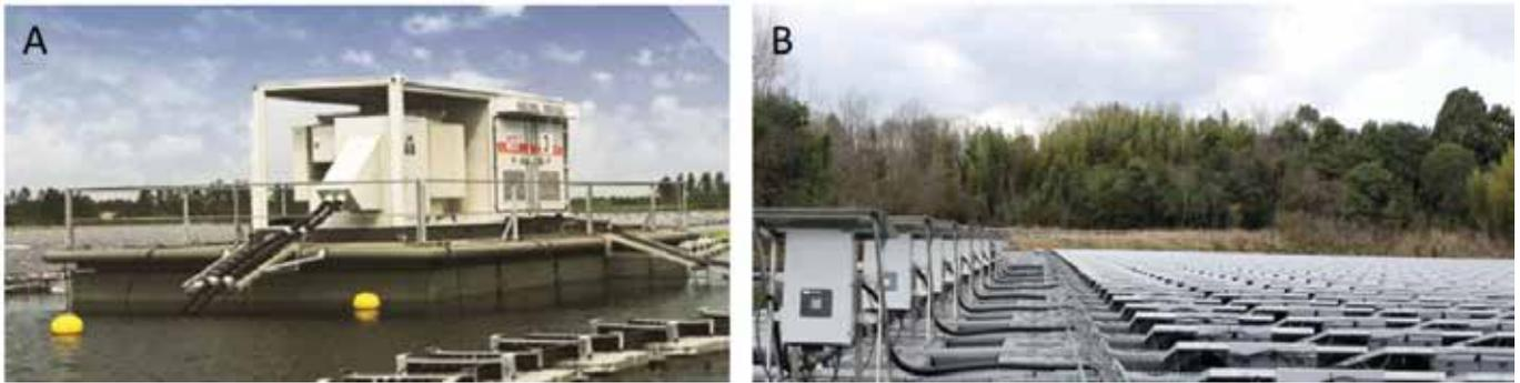
**Figure 3:** (A) Central inverter placed on floating platform at China. (B) String inverter
