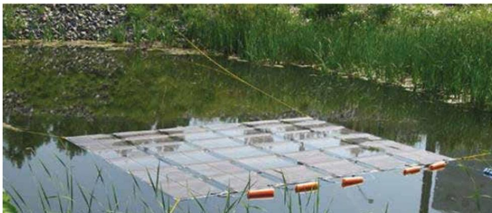
**Figure 18 :** 0.57 kWp submerged floating solar PV based plant
