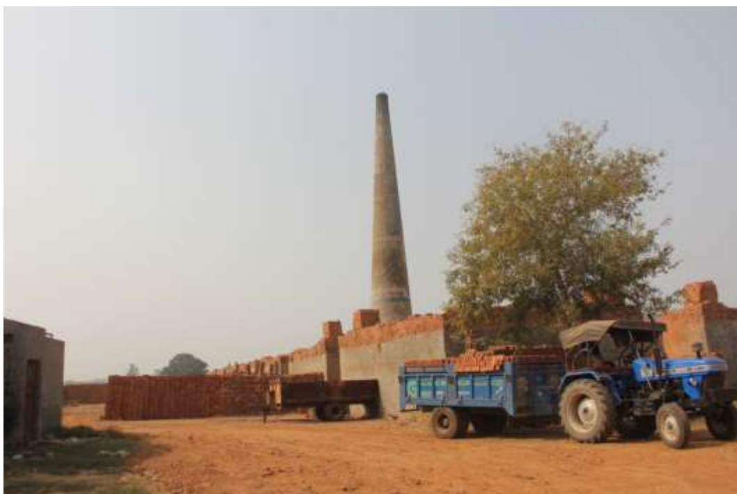
A brick kiln unit
