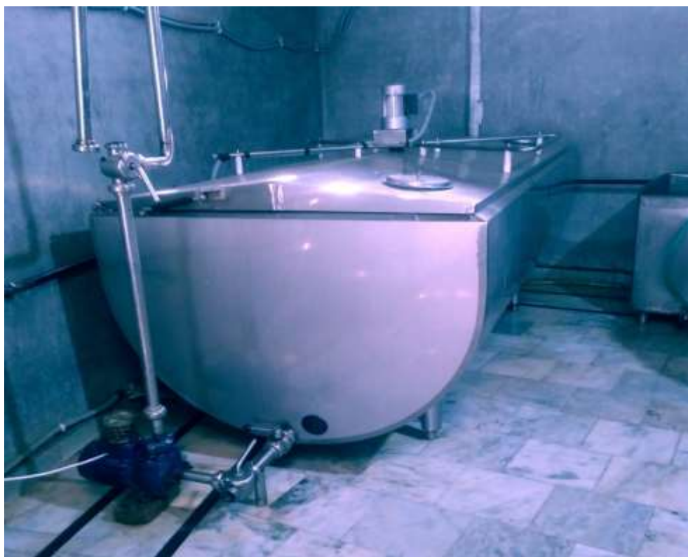
Bulk Milk Chiller
