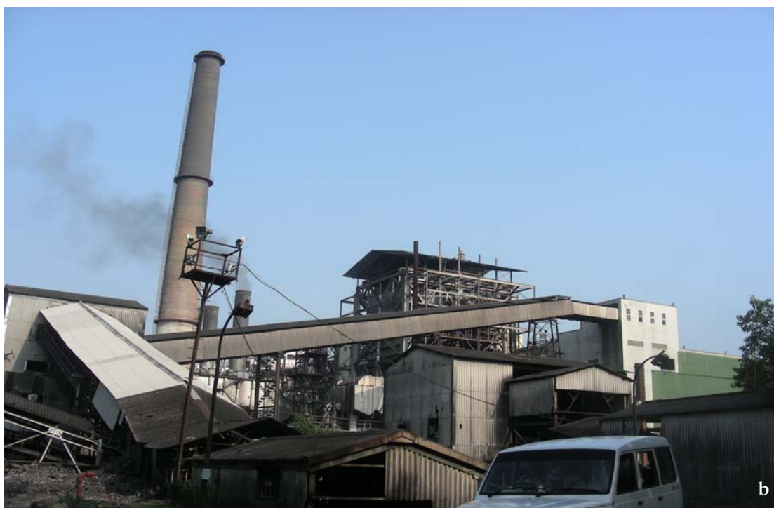
Plate 1 : Emission of black smoke from Kolaghat Thermal Power Station (6 x 210MW) (a), Bandel Thermal Power Station (4 x 80 + 1 x 210) (b)
