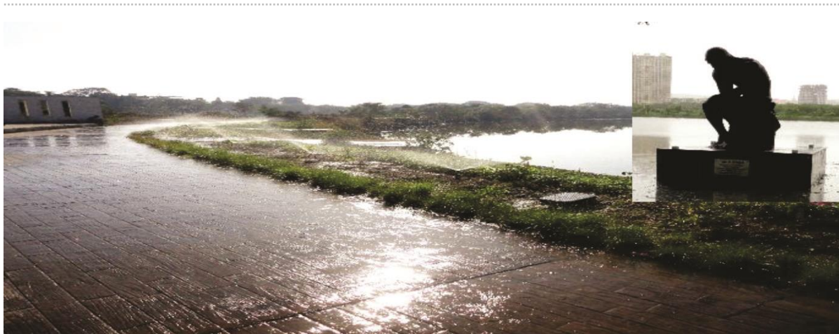
Picture No. 9: Water body at Nerul after its renovation and beautification
