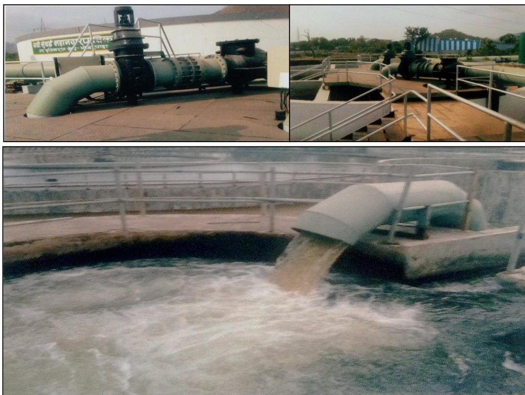
Picture No. 11: Back flushing of water at Bhokarpada water treatment plant
