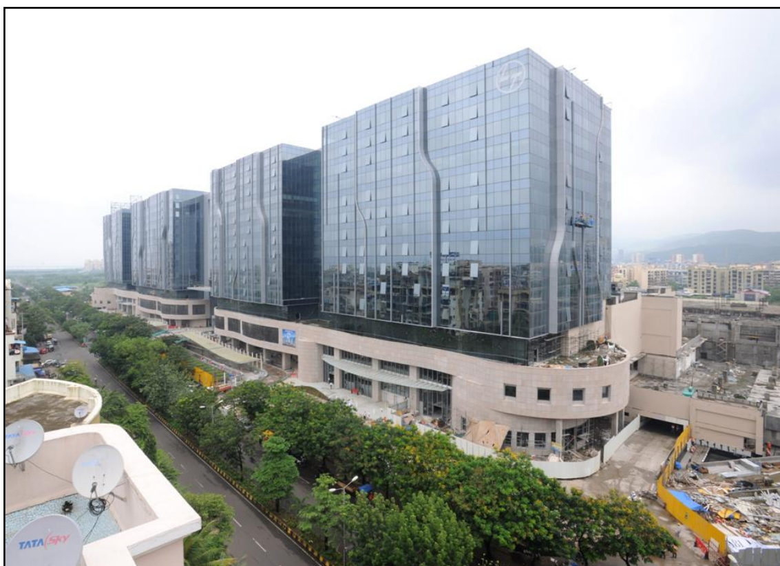
Picture No. 6: The partially completed Seawoods Grand Central Station
