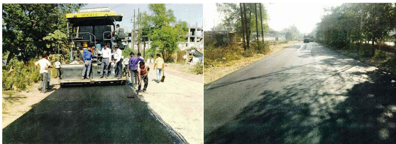
Picture No. 19: Road construction using Plastic waste at Turbhe MIDC
