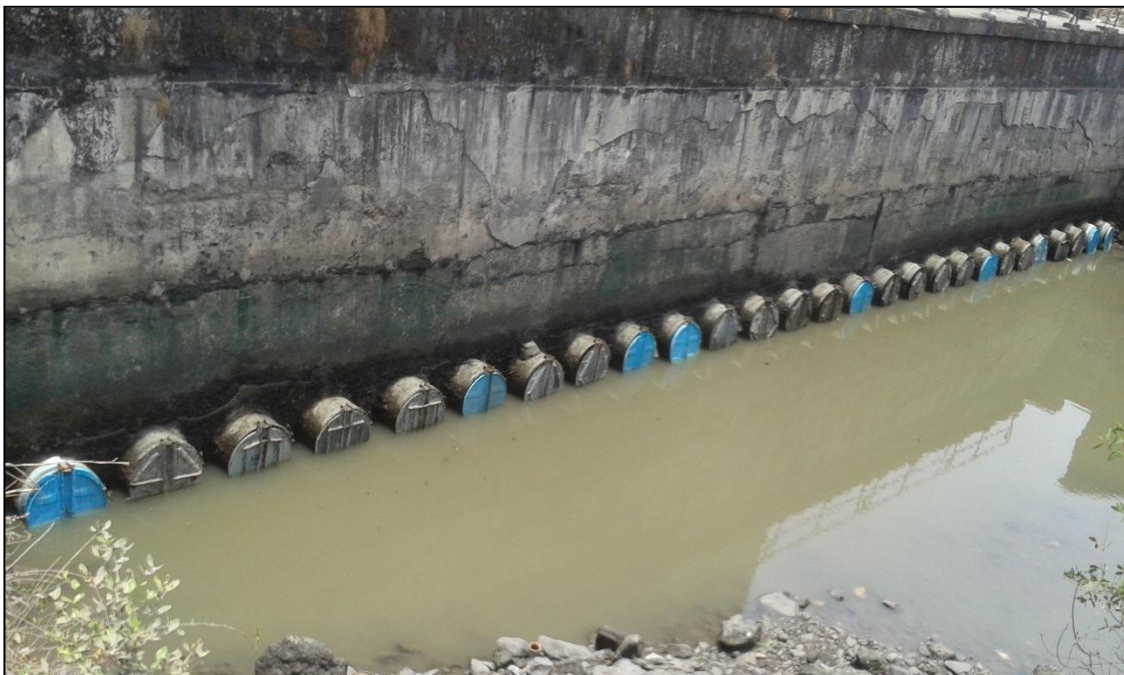
Picture No. 5: Dutch dyke (Holding ponds) with flap gates
