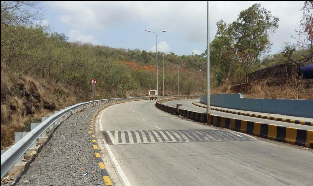
Picture No. 4: Completion of roads at MIDC
