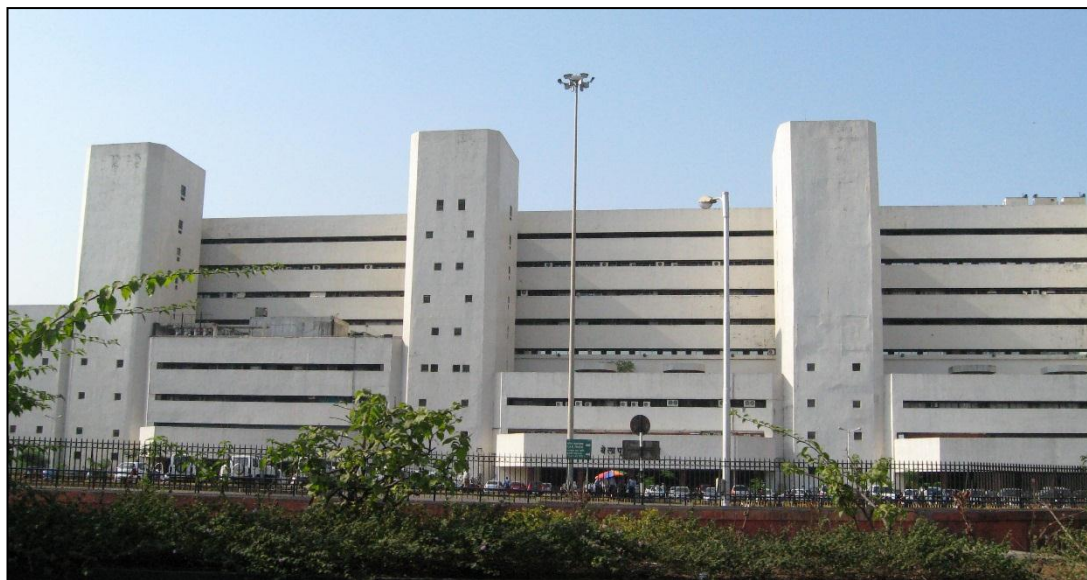
Picture No. 2: Belapur railway station complex
