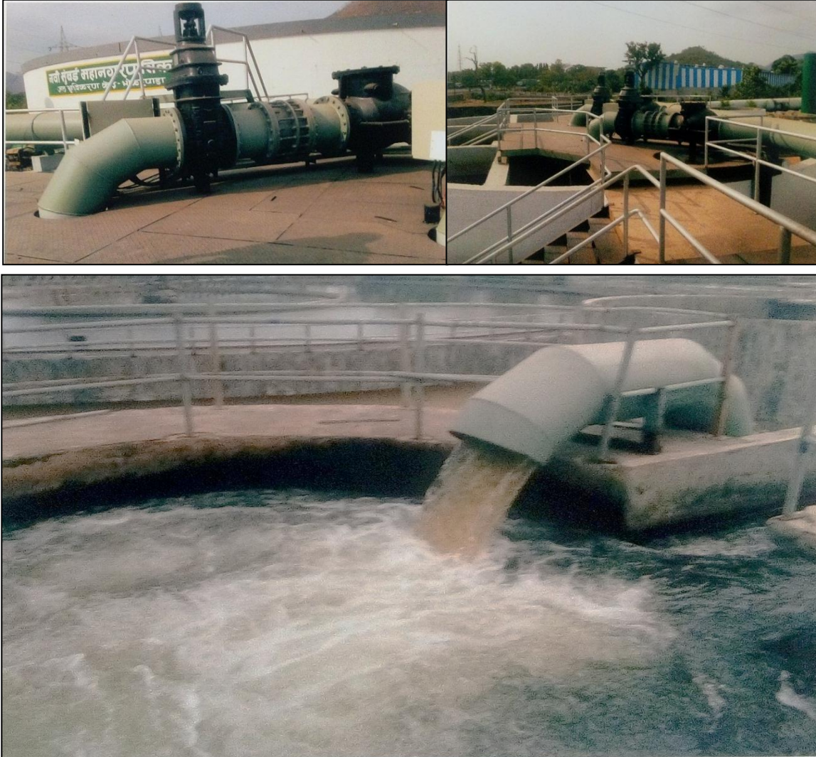
Picture No. 8: Back flushing of water at Bhokarpada water treatment plant
