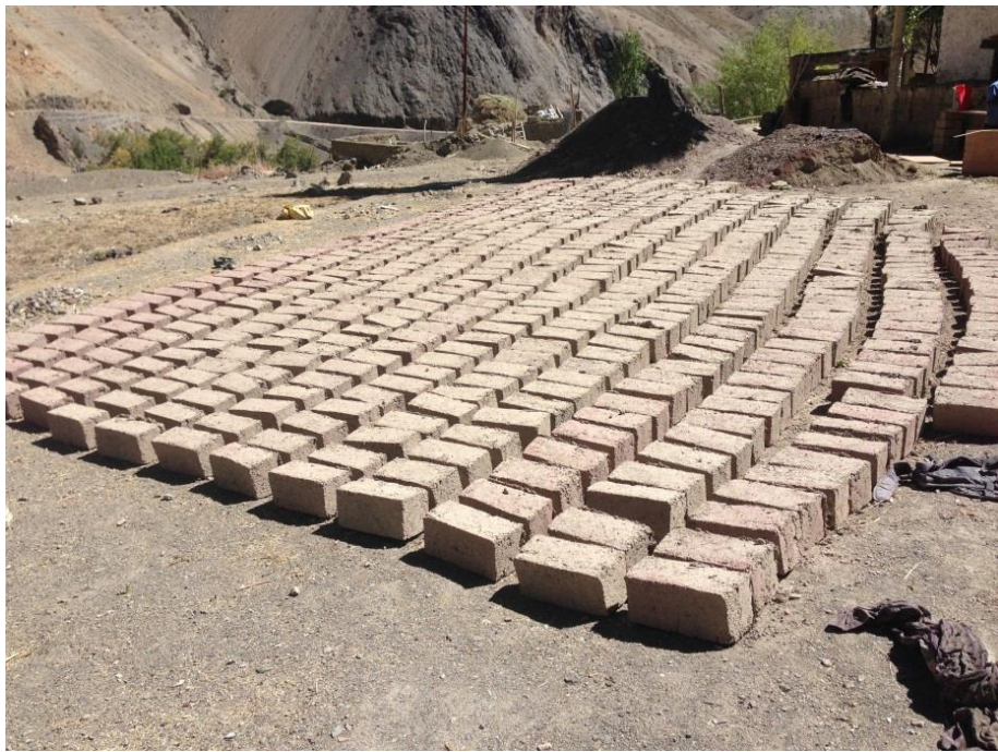
Figure6.5: Sun dried bricks being made on site.
