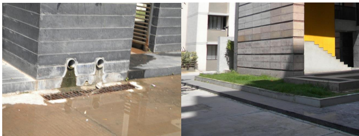
Figure 7.36: Storm water drains
