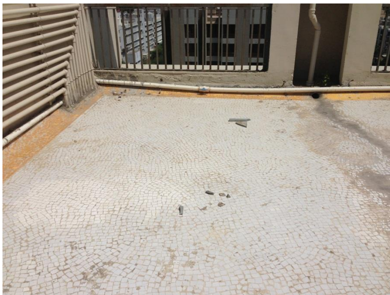
Figure 7.32: Roof finish in Solaris project
