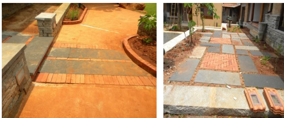
Figure4.5:Paving with mud concrete, brick and Cuddapah and sadaralli stones
