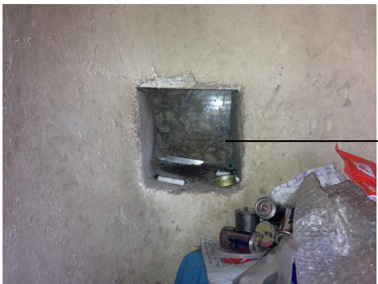
Figure6.6: A cut through section of wall showing saw dust used as insulation material.
