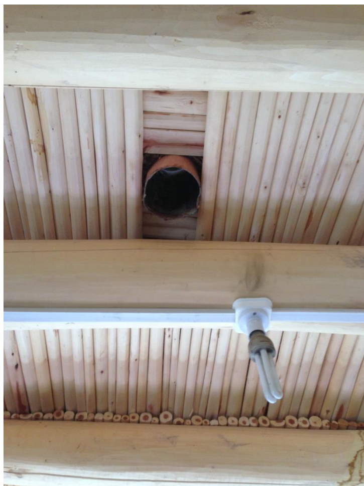
Figure 6.4: Typical roof construction from inside the house.
