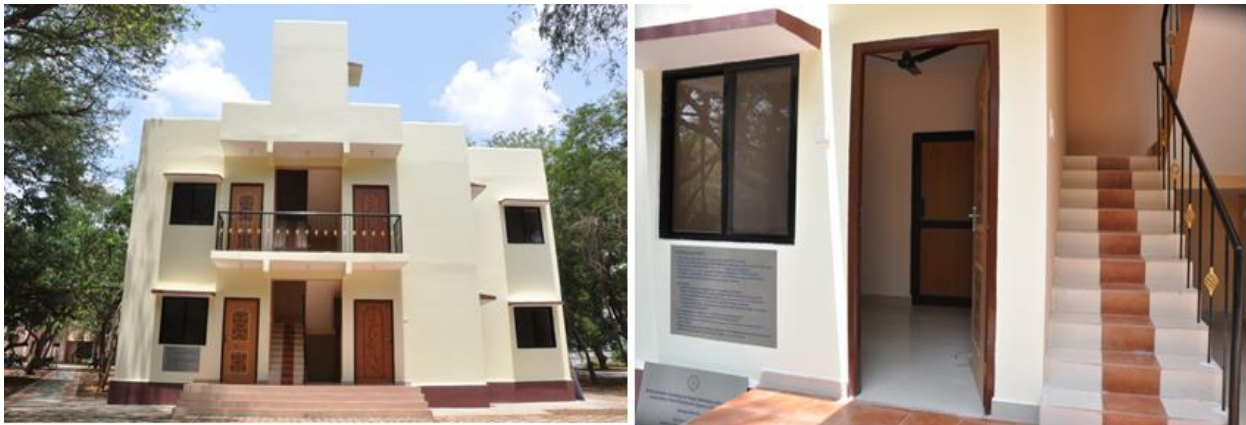
Figure3.10: Pictures showing the completed house at IIT Chennai7
