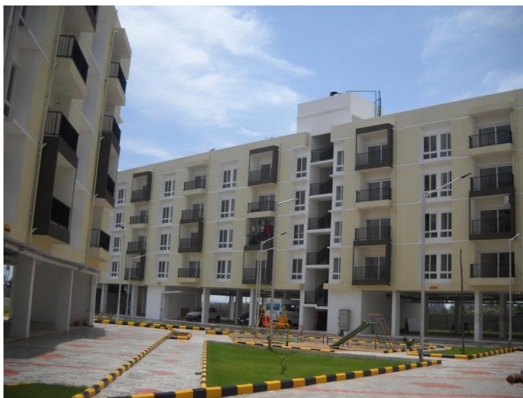
Figure5.1: A view from courtyard of the VBHC Housing
