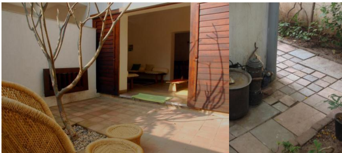
Figure7.8: Nimaj stone and waste brick paved pervious surfaces
