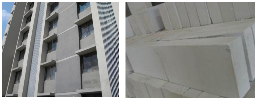
Figure 7.31: Autoclaved aerated concrete masonry wall for external wall
