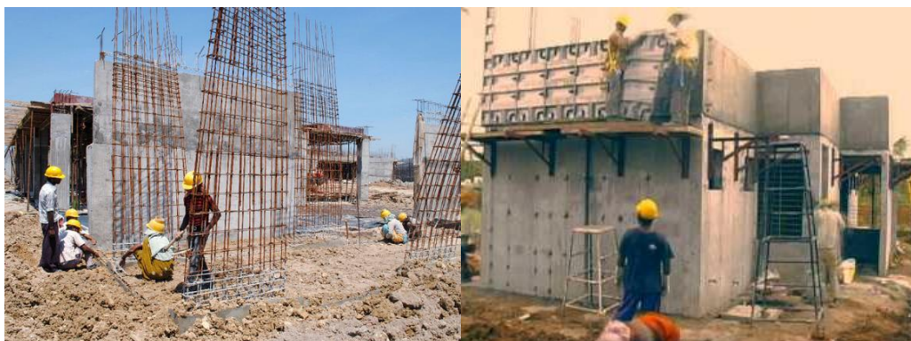
Figure 5.4: Construction of Reinforced Concrete (R C) wall
