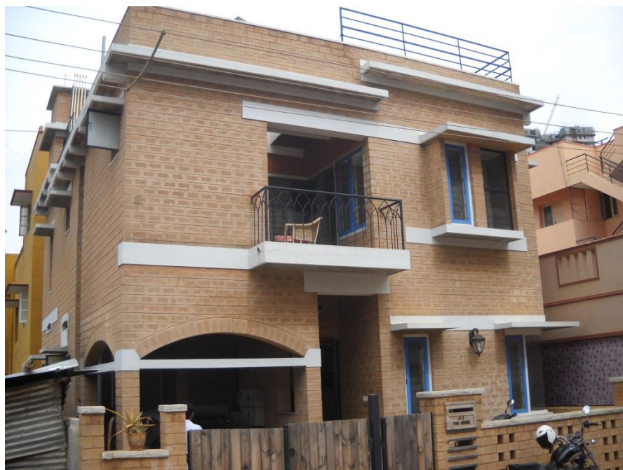
Figure4.32. Front view of Rohan & Reshmy's house
