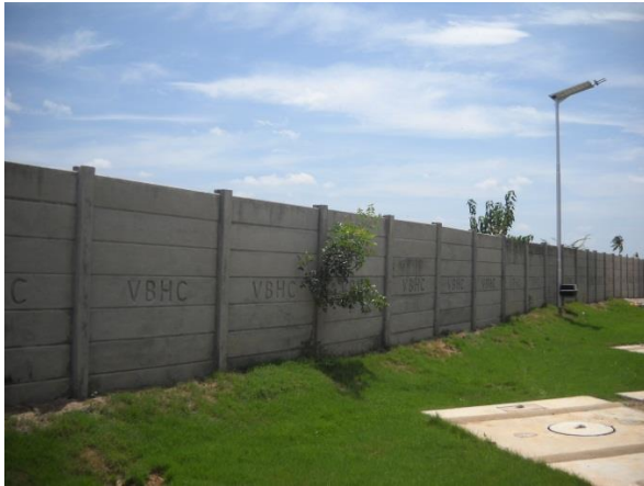
Figure5.5: Precast concrete slabs used for compound wall
