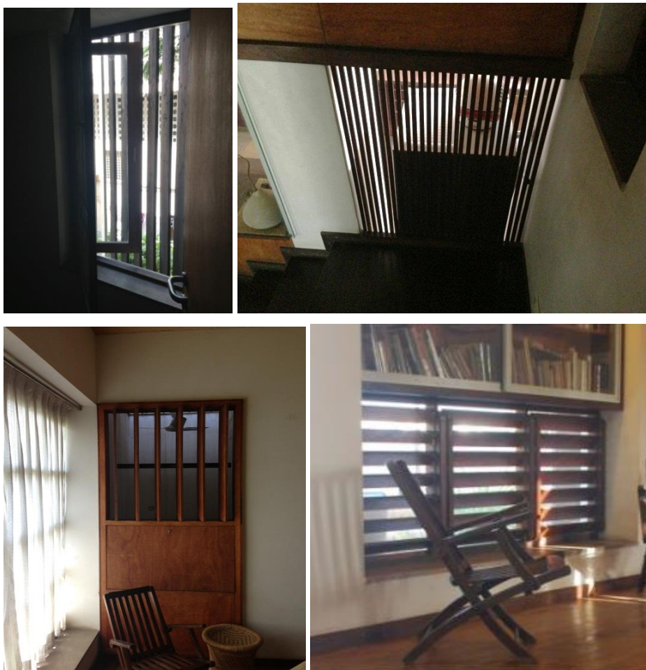
Figure7.17: Clockwise: Wind catcher outlet, external louvers to provide privacy and direct ventilation, internal ventilation openings between kitchen and staircase, window louvers system to open natural ventilation while controlling direct sunlight
