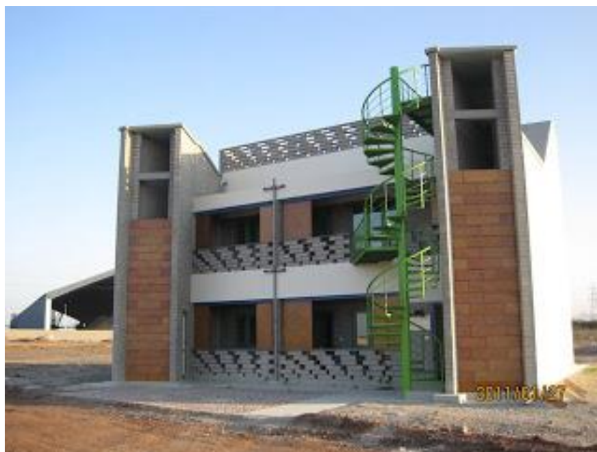
Figure3.14: A completed and Occupied Unit of the Project
