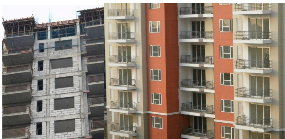
Figure8.10: During and after construction images of AAC block walls
