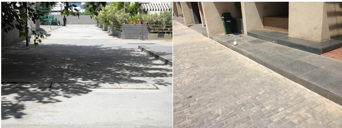
Figure 7.30: High SRI PCC pavement and interlocking concrete pavers
