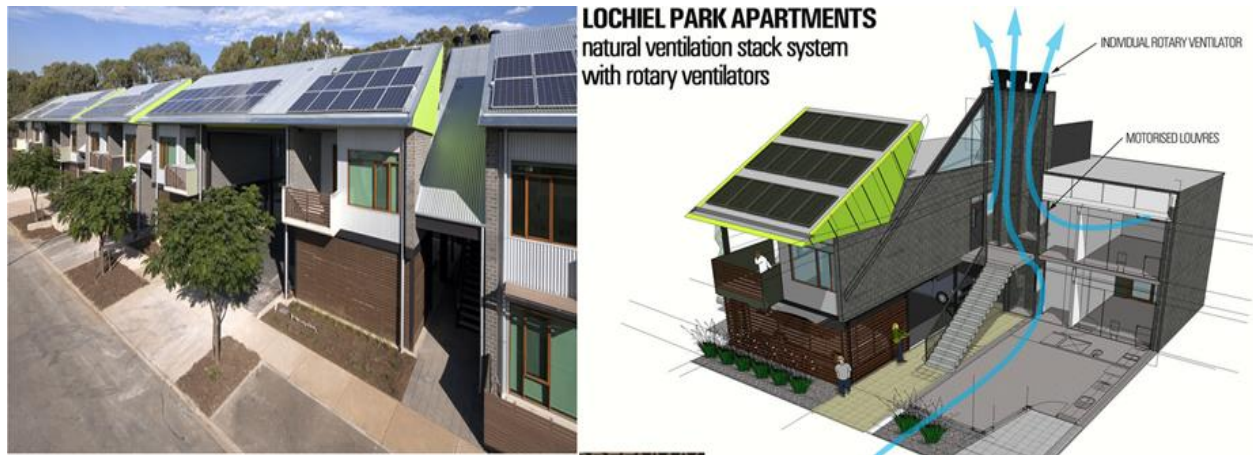
Figure 3.19: Left figure shows houses in Lochiel Park and in right the picture shows ventilation system concept used in houses
