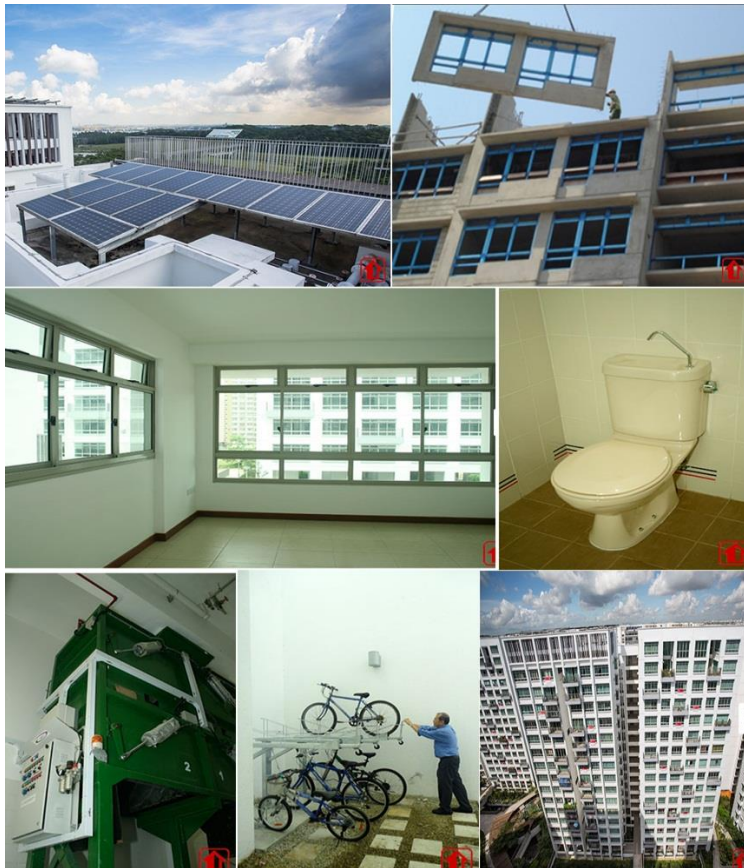
Figure3.16: Top left is picture showing solar panels being integrated on roof. Top right picture shows pre-cast technology. Middle left picture shows provision for natural lighting and ventilation. Picture on middle shows Eco-pedestal used to reuse water. Bottom left is the picture of centralised chute for waste collection. The cycle parking provision is shown in bottom middle picture. Bottom left is the building picture showing white outer self-cleansing paint
