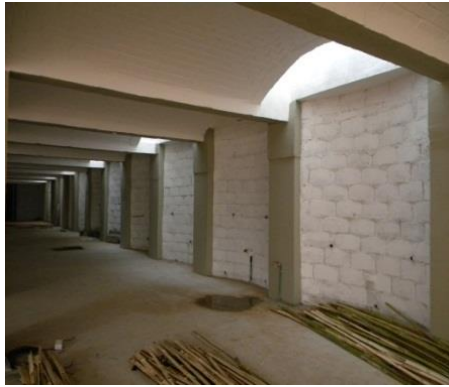
Daylight through roof in parking
