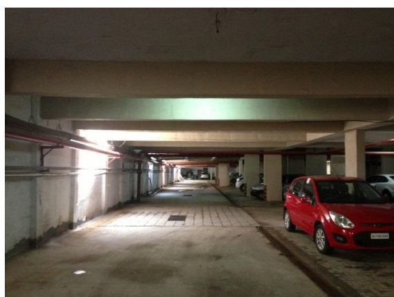
Figure 7.34: Photograph showing day lighting in basement parking area.
