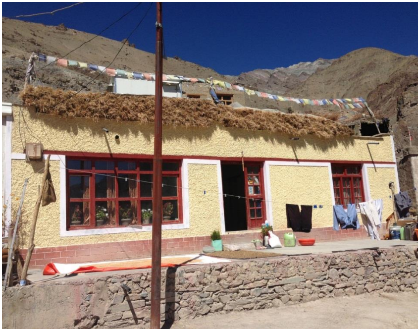
Figure6.7: DG house surveyed in the study.
