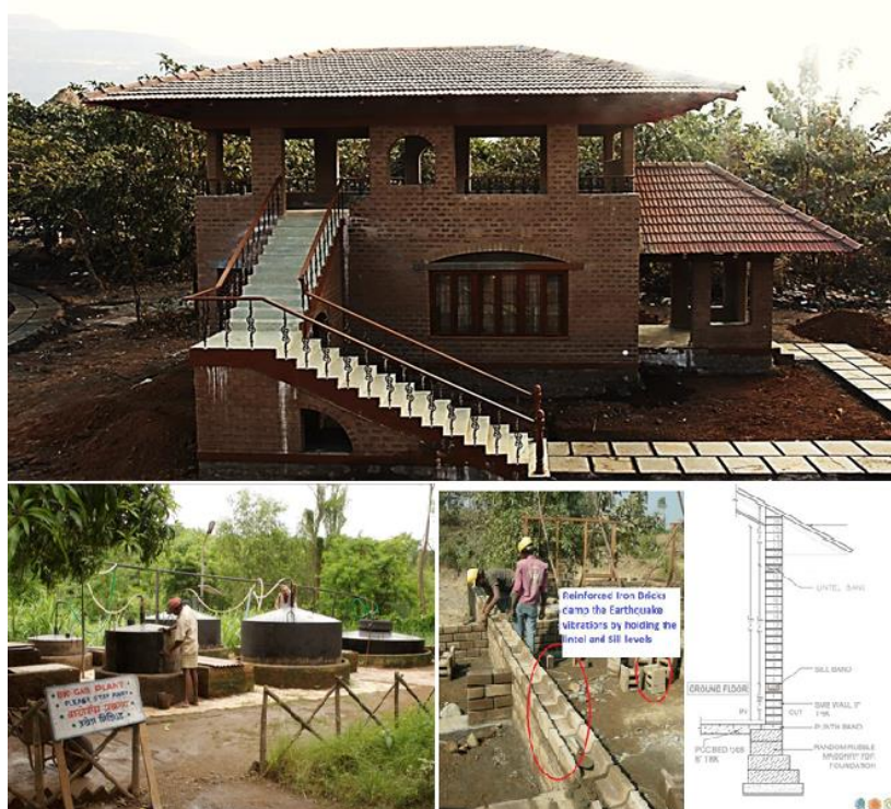
Figure3.11: Picture at top shows a completed house. Bottom left picture shows bio-gas plant installed in the village. Figure on bottom left shows worker constructing walls made of special bricks
