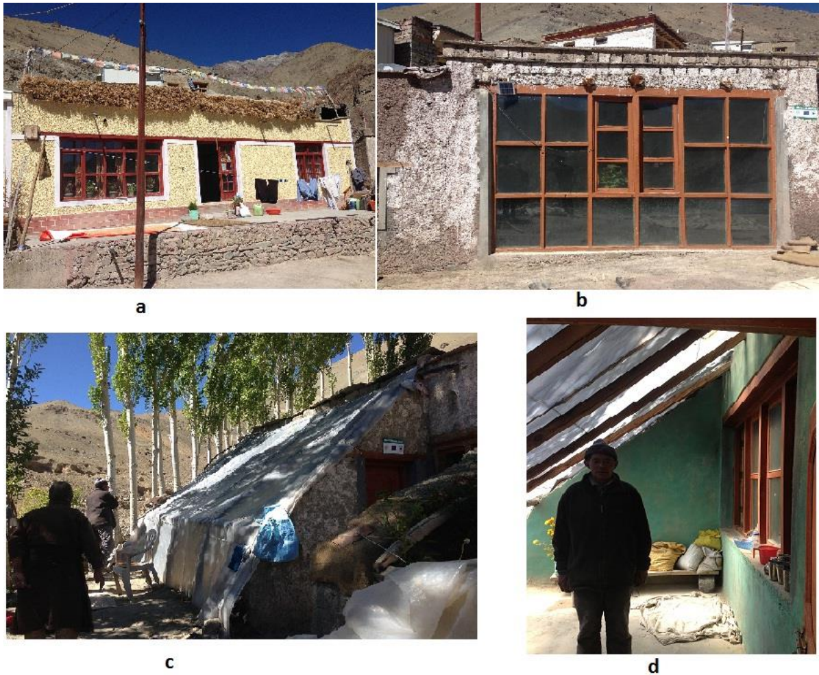
Figure 6.2: a) A direct gain house, b) House with Solar wall, c) Attached green house to the house, d) Inside of a green house.
