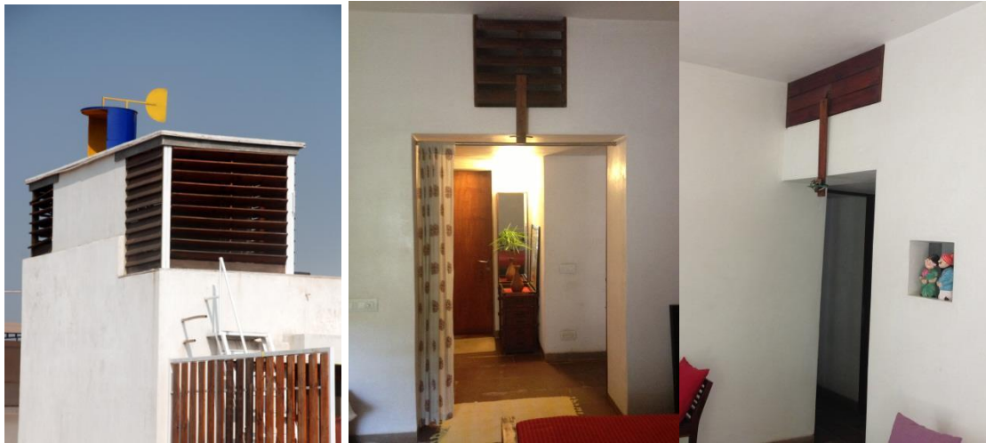
Figure 7.20: Left: Cooling tower inlet, middle & right: Tower outlets
