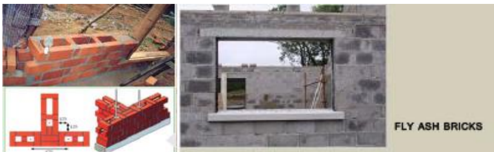
Figure7.45: Rat Trap Bond (Left) and Use of Fly ash Bricks (Right)
