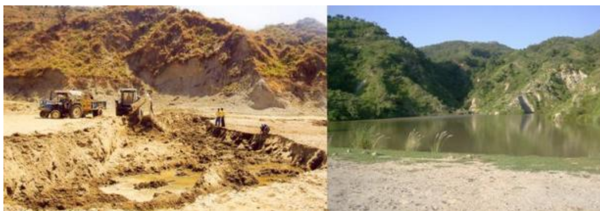
Photo 4 Shiv Mandir dam at Jhanda during desiltation, and filled with water after desiltation
