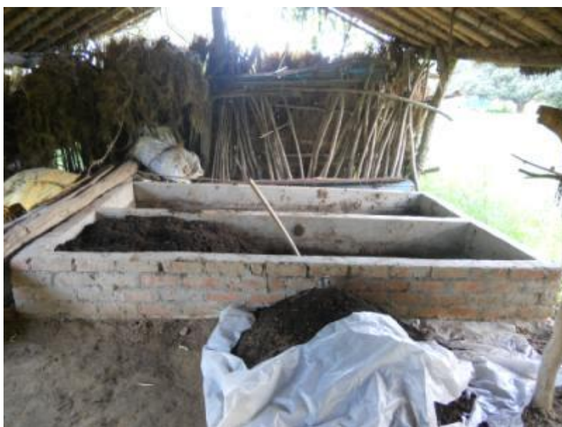
Photo 5 Vermicompost pit during construction
