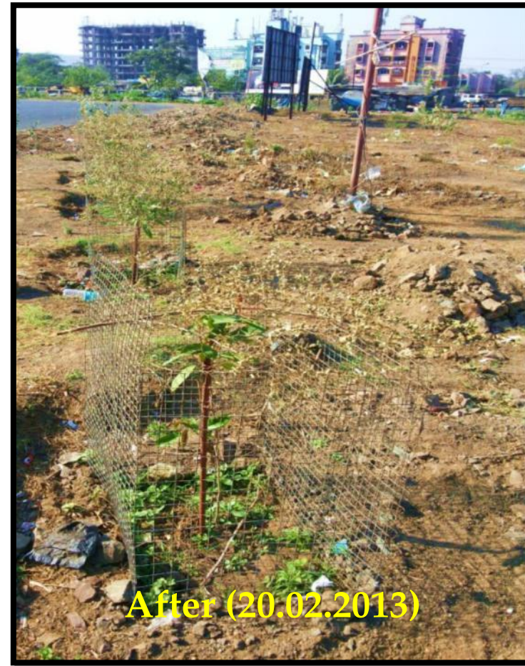
Picture No. 35: Installation of tree guards and thorny bushes for protection of the plants from grazing animals
