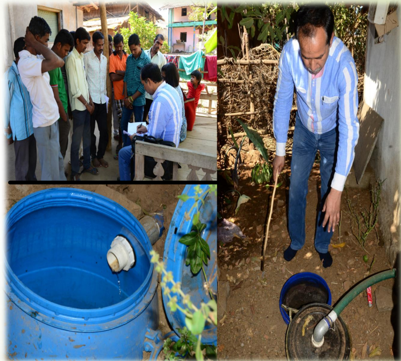
Training and demonstration- Installation of the grey-water treatment system
