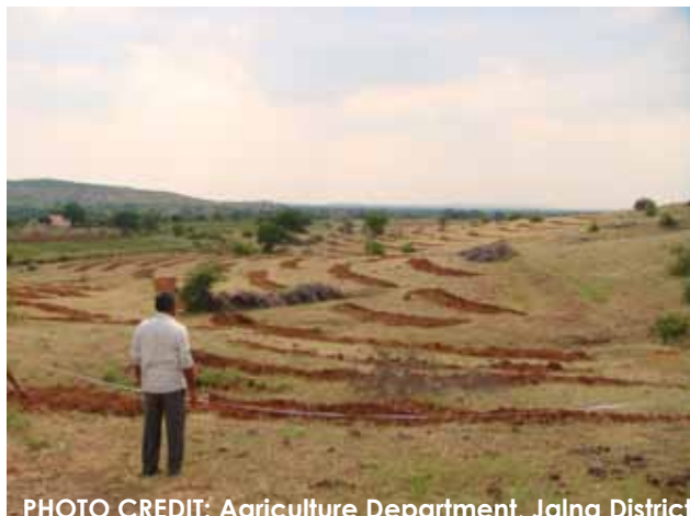
PHOTO 6.2 Contour Trenching carried out in Kandari, Jalna, in June 2013
