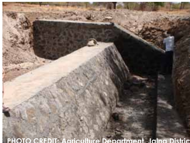
PHOTO 6.3 Community Nala Bund, Badnapur, Jalna, constructed in June 2013
