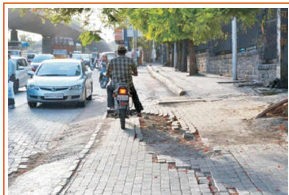
Photo 1: Use of cycle track by motorist
