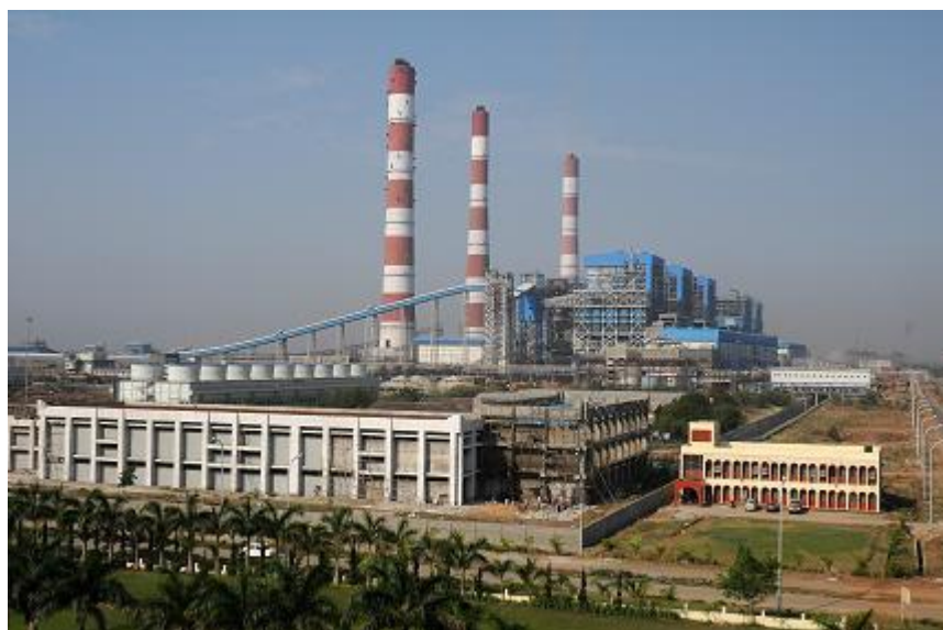
Figure 5 Sipat thermal power station, NTPC
