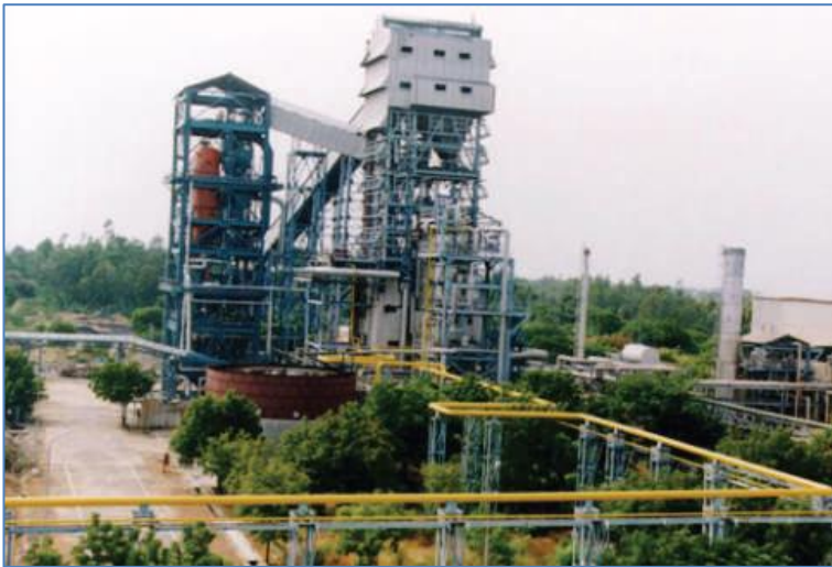
Figure 8 BHEL IGCC development facility at Tiruchirapalli (6.2 MW)
