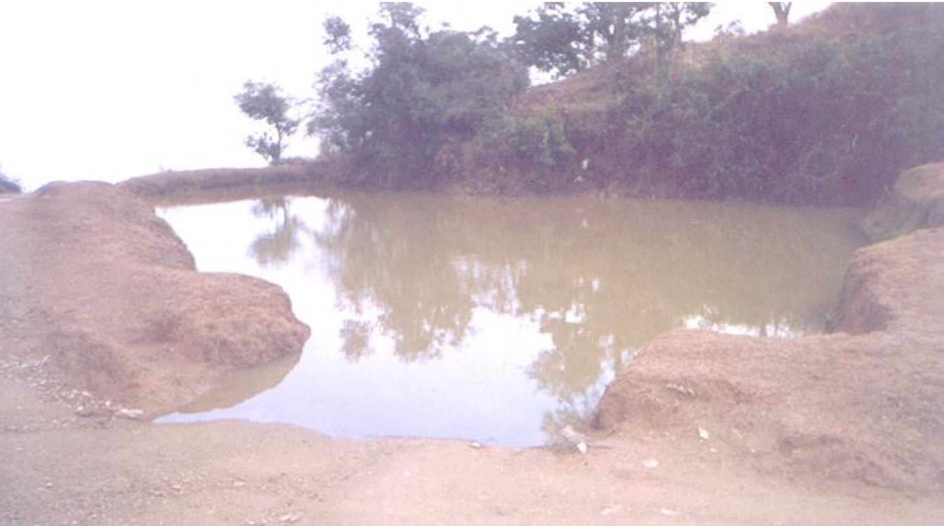
View of a traditional Chahal (recharge pit)
