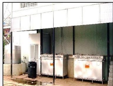
Installation of Bio-methanation Plant at NMMC HQ (May 2014)
