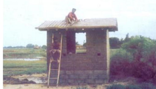
Installation of bamboo reinforced soil roof. (Source: Bhubaneswar Lal Shrestha)
