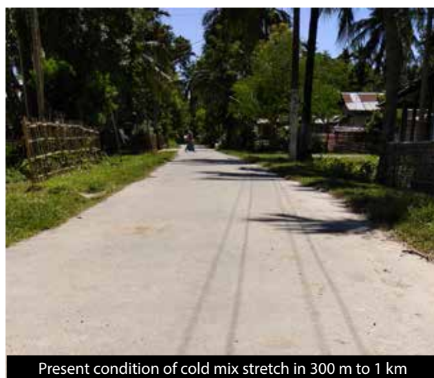
Figure 34 Present condition of sample rural road project using cold mix
