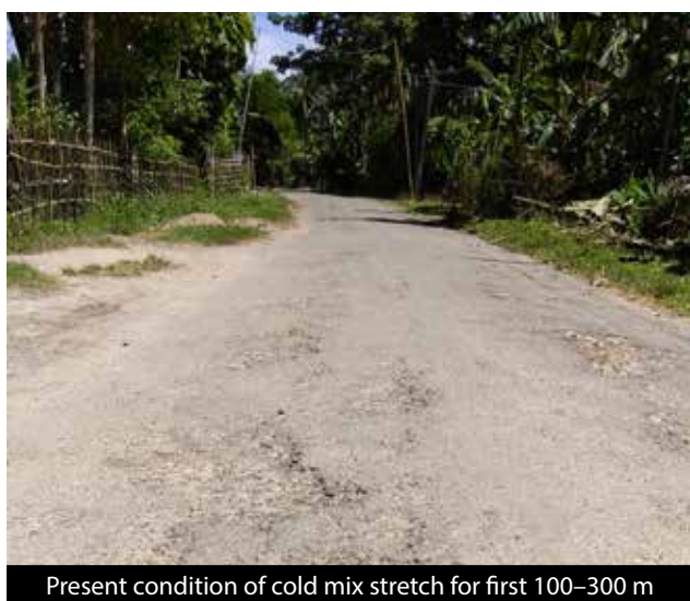
Figure 34 Present condition of sample rural road project using cold mix
