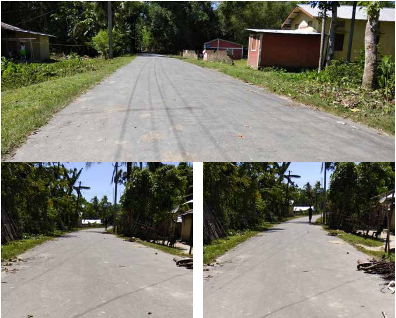
Figure 35 Present condition of sample rural road project using hot mix
